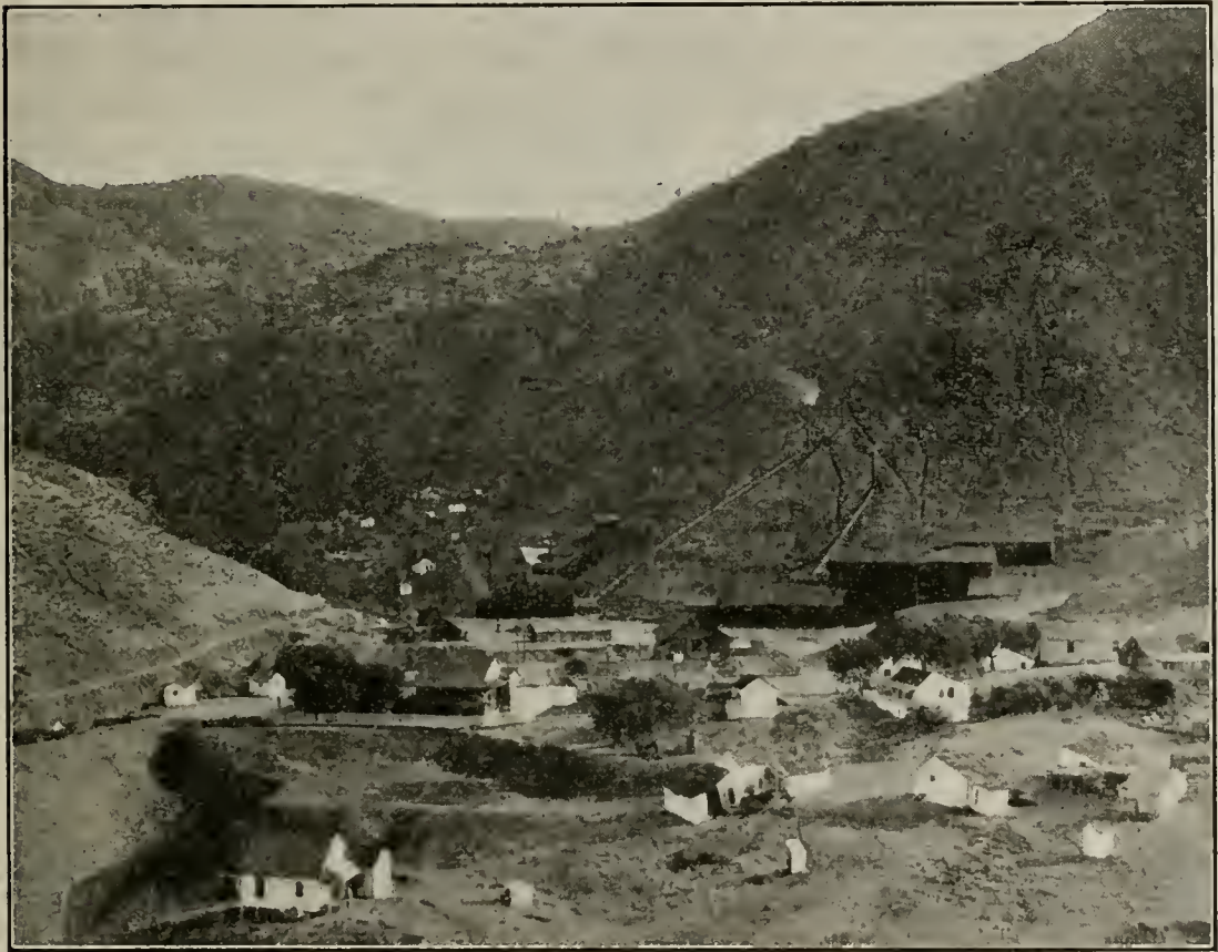
The New Idria Quicksilver Mine, San Benito County, California. The largest quicksilver producer in the United States.
